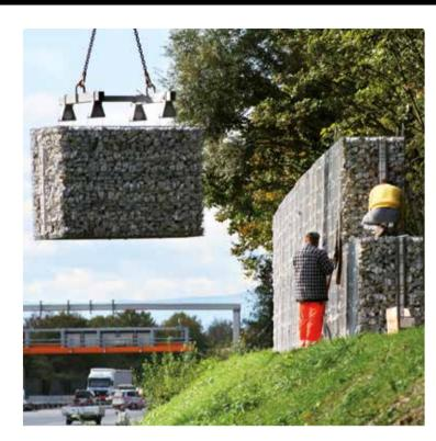
Gabions that are only filled with stones do not provide effective noise protection. To fulfil the noise protection specifications in the relevant standards, it is necessary to install a noise-protection core in the stone basket
