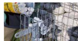
After construction, the fence gabion is filled from above.
