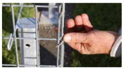
An exact-fitting spiral wire ensures precise corner joints.
